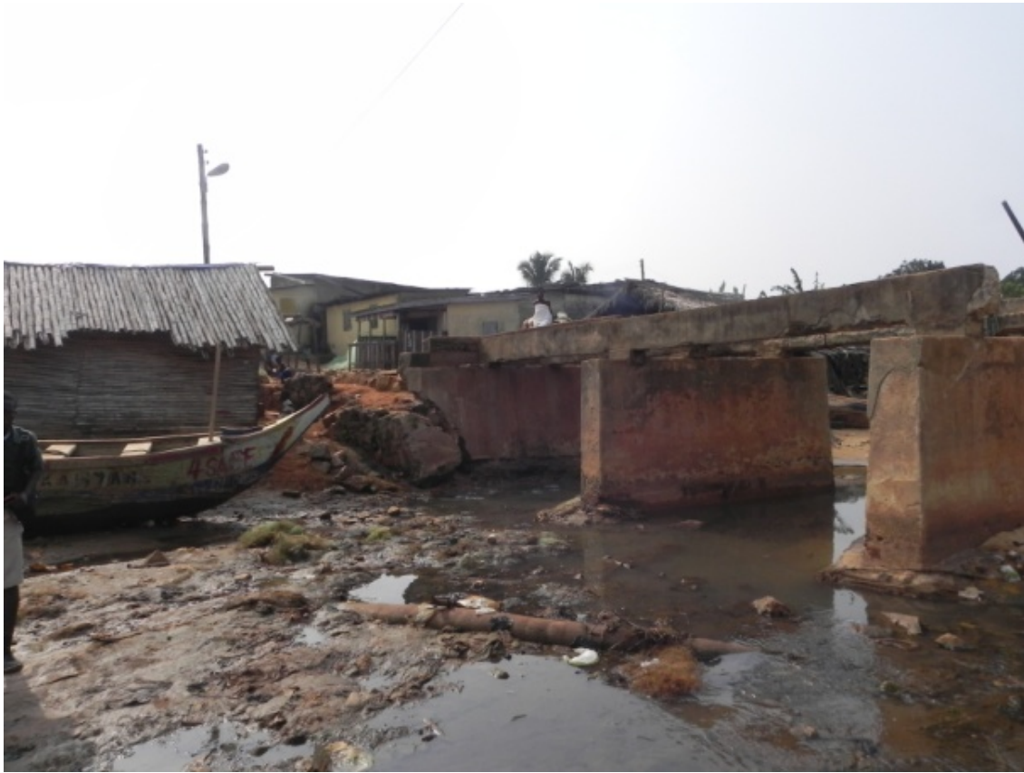
Figure 16 Damage to coastal infrastructure in a coastal settlement in Nzema East indicates ongoing problems from erosion and flooding
